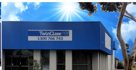
VIC Office & Manufacturing
